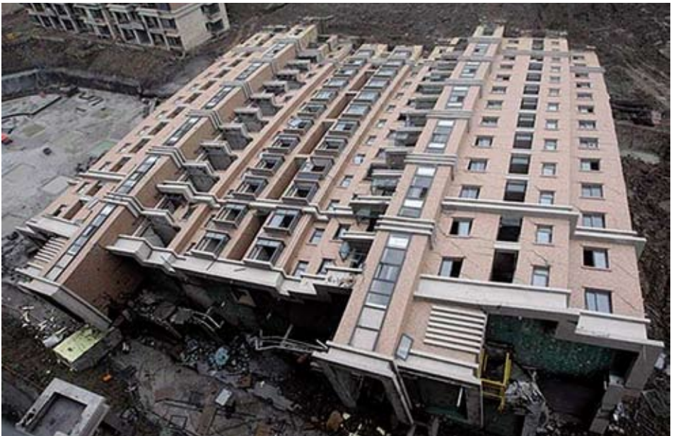
On June 29 2009 the 13 storey Lotus Riverside apartment building in Shang-hai's Minhang district collapsed killing a 28-year-old worker surnamed Xiao. The building was under construction, the developers' construction licence had expired in 2004.
